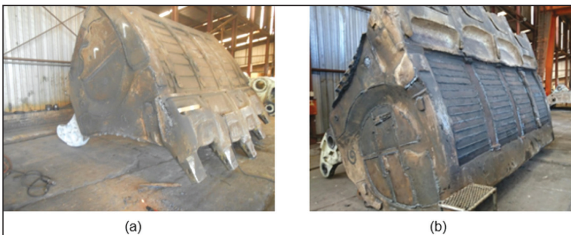
FIGURE 3: Stripping and gouging components before repair: (a) Component relined with AR-Plates (b) Component relined with CCO (JCB-Gearvest (Pty) Ltd, 2018)
