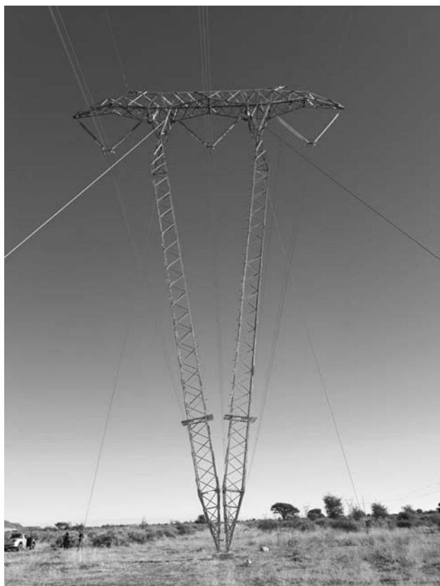
FIGURE 1: A type 520B guyed V-tower
